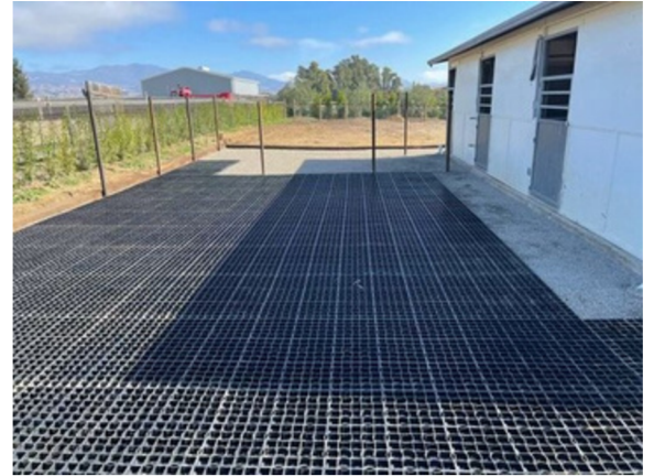
Livestock holding area reinforced with ARW Ground Grid, improving drainage and reducing mud during wet seasons.
