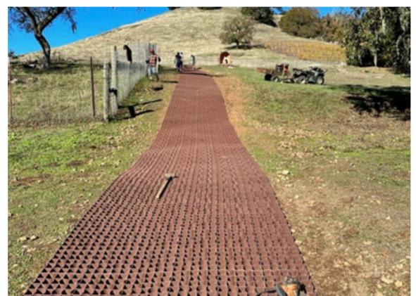
Slope access track stabilised with ARW Ground Grid to prevent erosion and improve traction.
